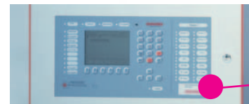
The flexible FMZ 5000 fire detection control panel monitors and controls the attached automatic extinguishing systems
